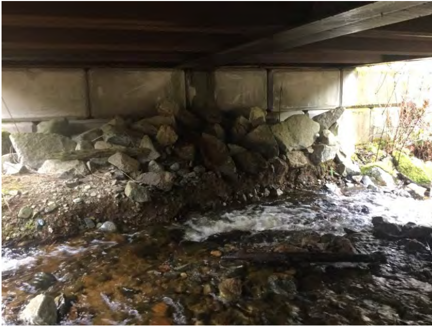
Left Bank Abutment when facing downstream
