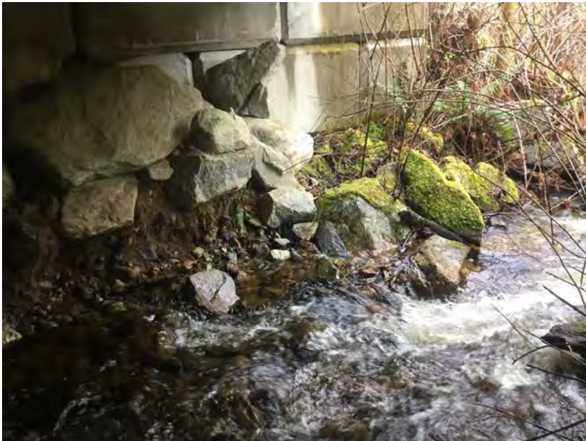
Left Bank Abutment when facing downstream
