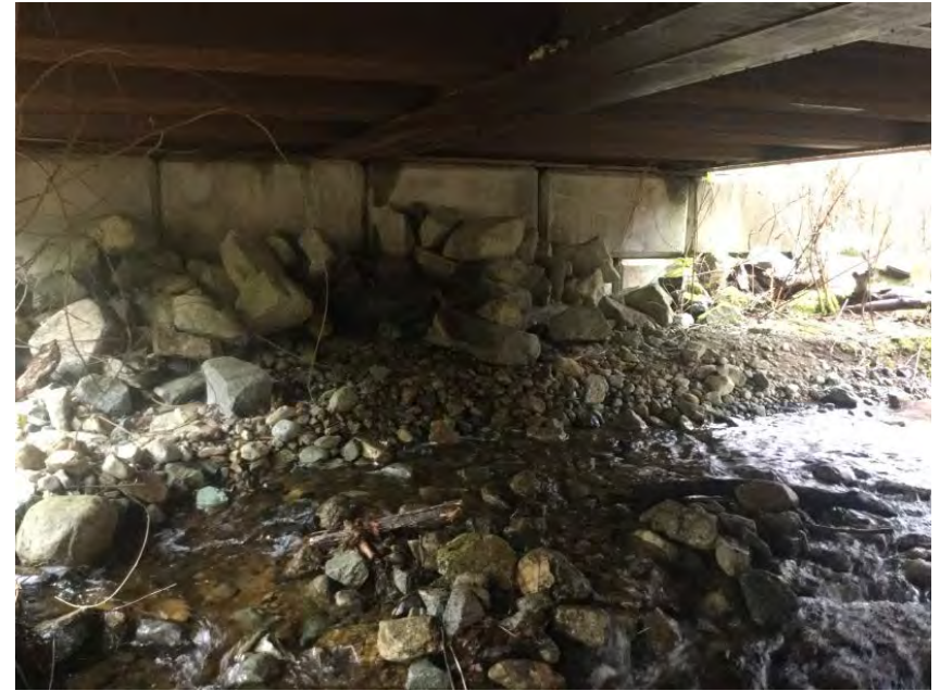
Right Bank Abutment when facing downstream
